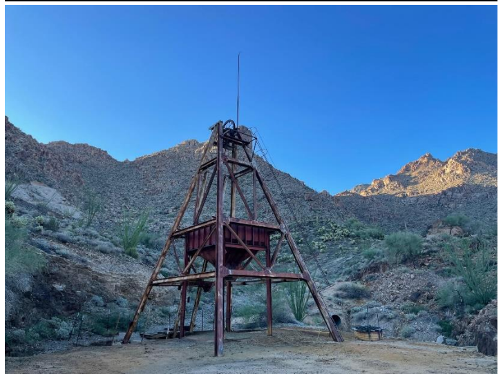
Figure 11: The historic headframe at Antler (looking northwest)
